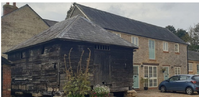
The Granary at Church Farm uses plank board as an external walling material.
