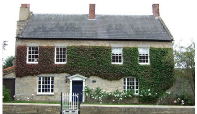
Grange Farmhouse, High Street
